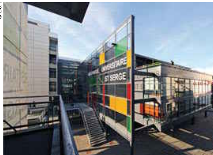
Angers. Saint-Serge. Pierre Pacault, Jean Collin, architectes.
